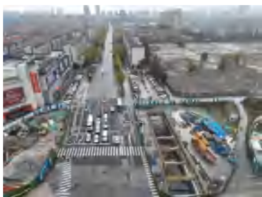
(81)钟秀路站附属施工防护 2022.11
