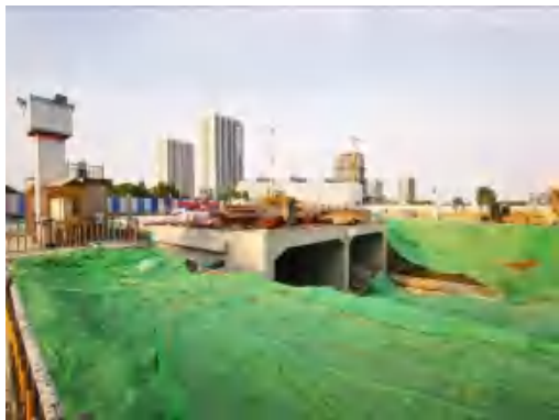
(141)通富路站裸露面苫盖 2021.6
