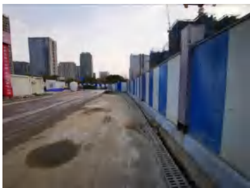
(51)永达路站新建排水沟 2020.12
