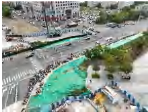
(62)永怡路站附属施工防护 2022.9
