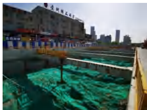
(108)五一路站裸土苫盖 2020.5
