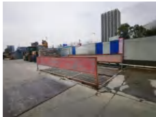
(142)通富路站洗车槽 2021.11
