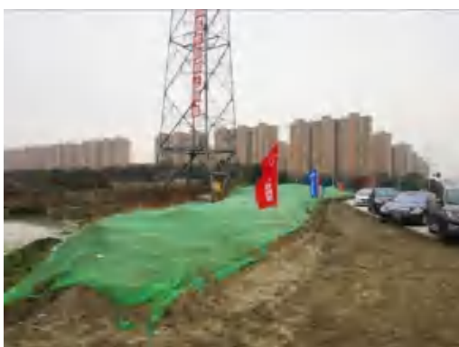
(27)幸福车辆段出入段线裸土苫盖 2020.12
