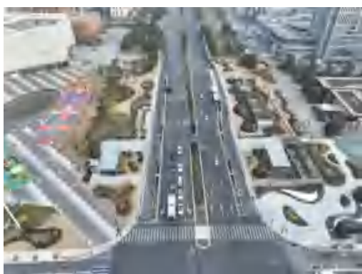
(145)通富路站绿化面貌 2023.12
