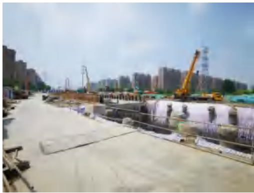
(29)幸福车辆段出入段线施工防护 2022.7
