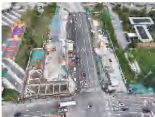
(143)通富路站施工面貌 2022.9
