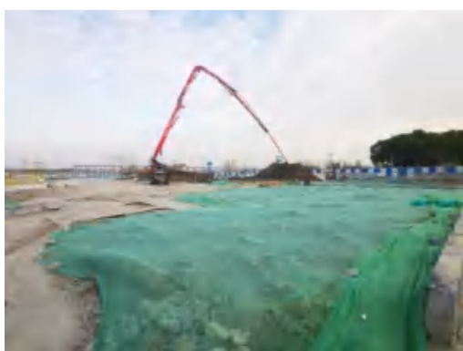
(169)南通东站裸土苫盖 2021.12
