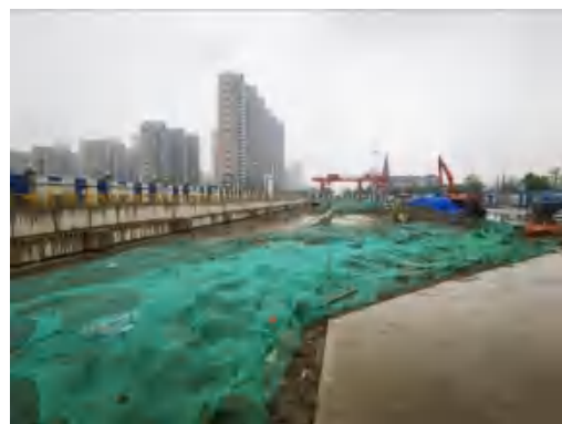
(116)园林路站裸土苫盖 2021.4
