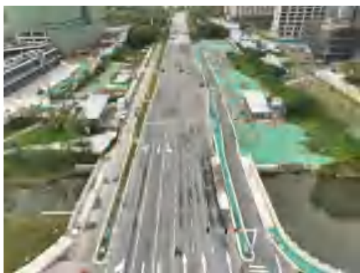
(55)永达路站场地恢复 2023.6
