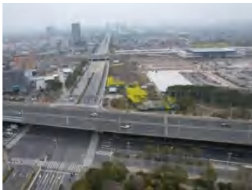
(174)南通东站绿化及场地复耕面貌 2026.3
