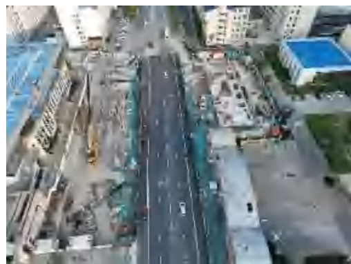
(110)五一路站附属施工防护 2022.9
