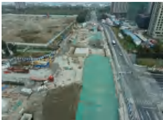
(53)永达路站道路恢复苫盖 2021.11
