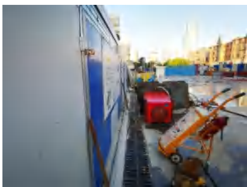
(97)易家桥站临时排水沟 2020.9
