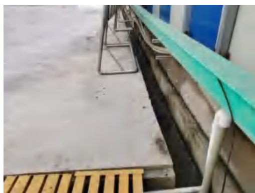
(34)幸福镇站临时排水沟 2019.12
