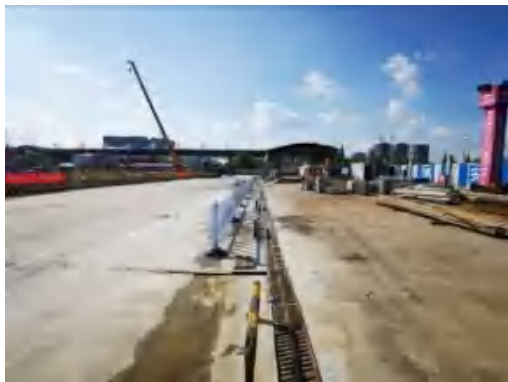
(45)南通火车站场地排水沟 2020.9
