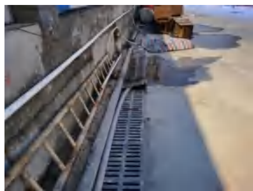
(68)北城大桥站临时排水沟 2019.12
