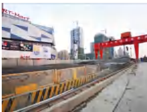
(60)永怡路站渣土坑 2020.12
