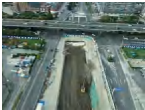
(69)北城大桥站基坑回填 2021.9
