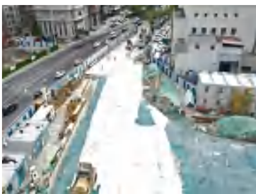
(99)易家桥站裸土苫盖 2022.6
