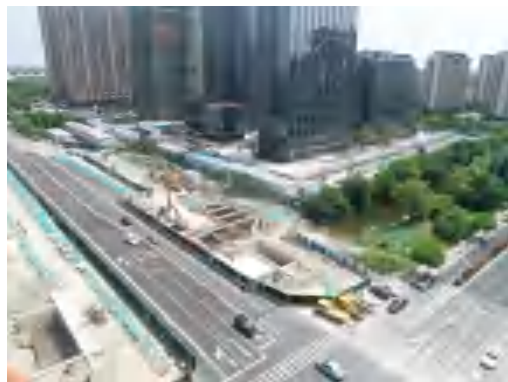
(54)永达路站附属施工防护 2022.5
