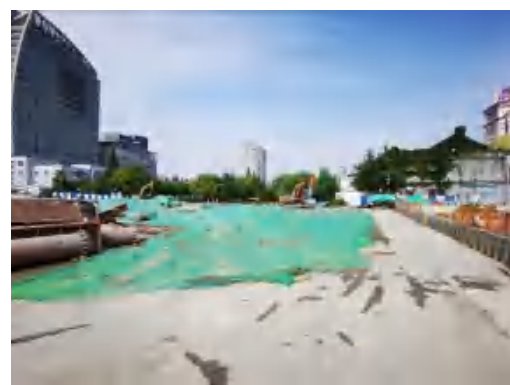
(90)体育公园站裸露面覆盖 2021.6
