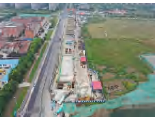
(115)园林路站施工面貌 2020.9
