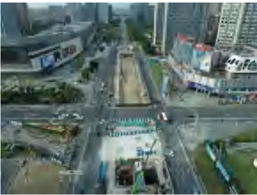
(61)永怡路站施工面貌 2021.9
